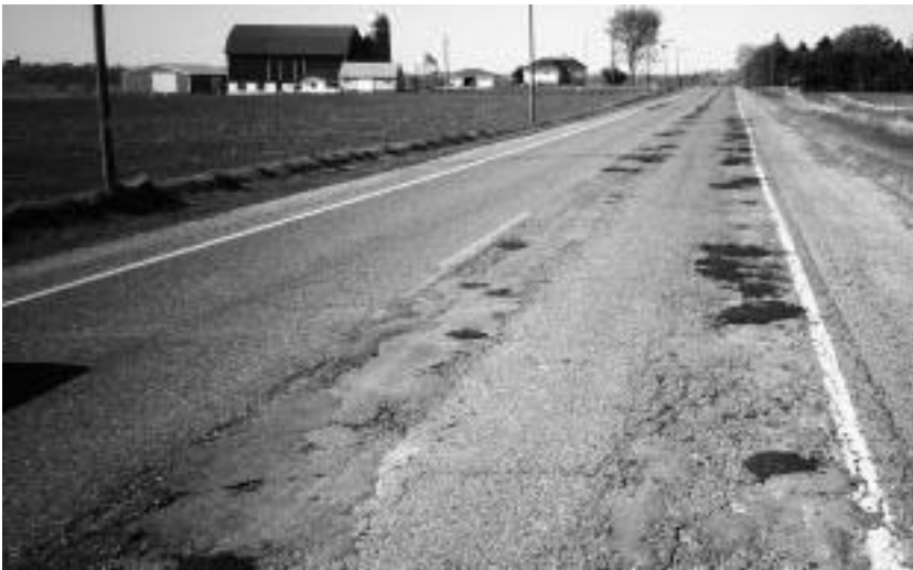
▲ Patches in poor condition, wheelpath rutting. Pulverize, strengthen and reconstruct.
