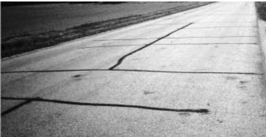
▼ Open crack, 1/2" wide; adjoining pavement sound.
