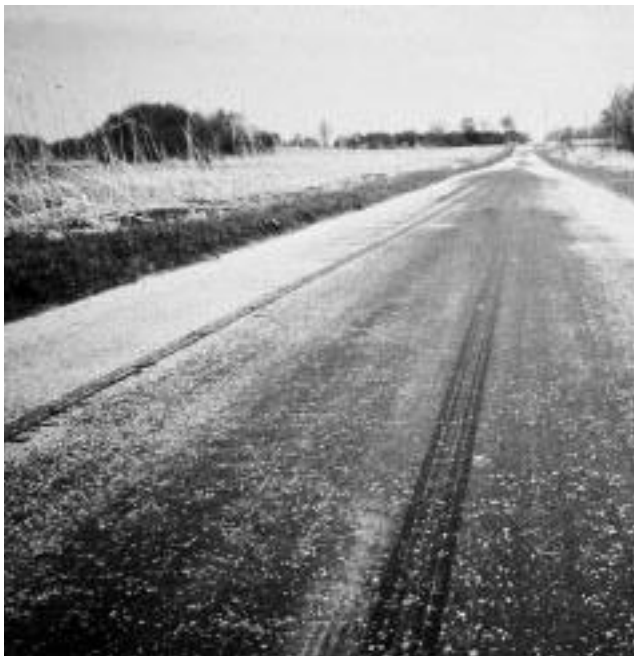
▼ Severe flushing.
