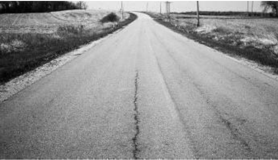
▼ Slight rutting; patch in good condition.
