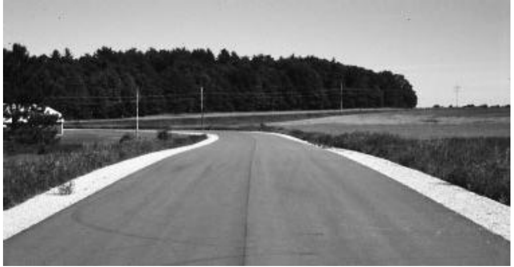
▶ RATING 10 New construction.
