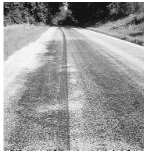
▼ Moderate flushing.
